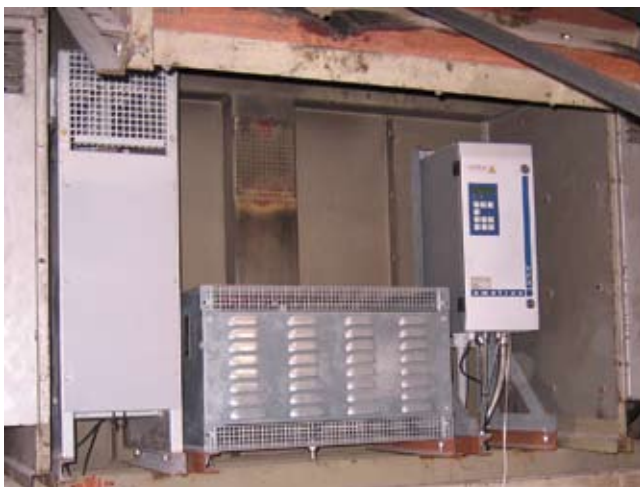
The retrofit involved installing a new electronic control system based on the Emotron VFX variable speed drive, as well as replacing the eight drive motors.
