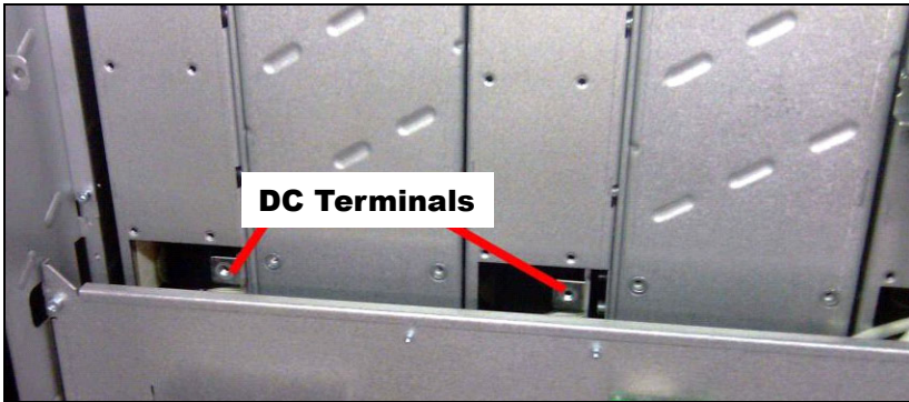
Fig. 2 Position of the DC terminals
